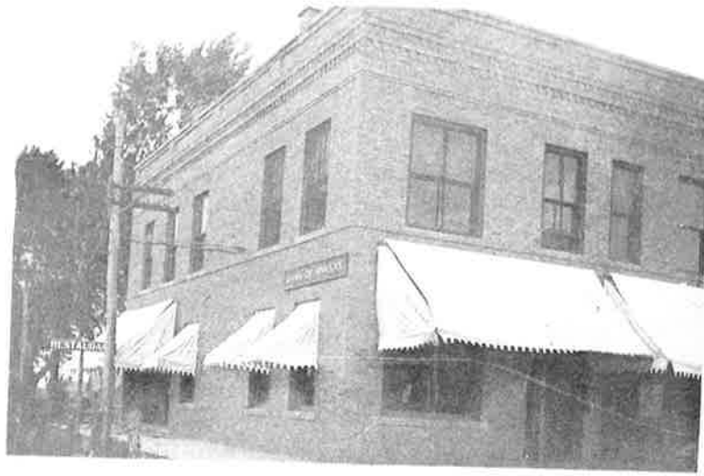
Bank of Ankeny - early 1900's (note: hitching posts and restaurant)
