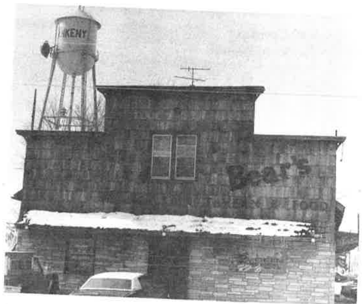
302 Maple Street built by Mr. Hallowell in approximately 1912
