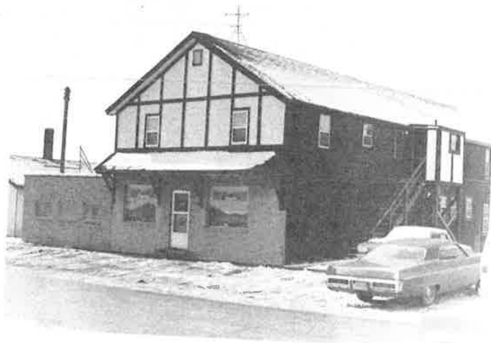
312 Maple Street built approximately 1910
