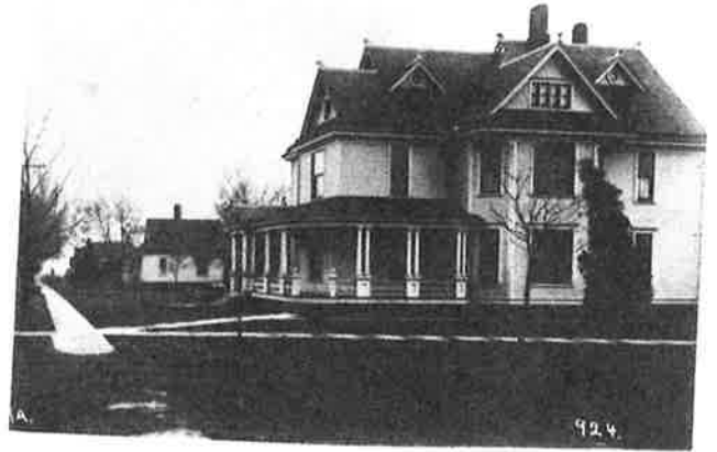
The Henry Wagner house, Third and Walnut Streets. (house was later moved to farm one mile north of Ankeny.)
