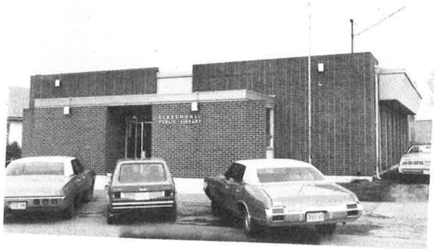
present facility on 211 S.W. Walnut Street
