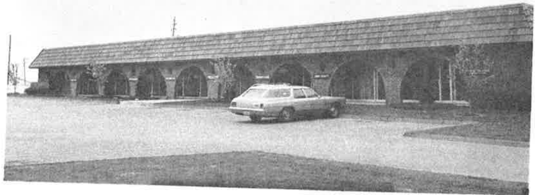
Ankeny Office Center N.E. Trilein Drive
