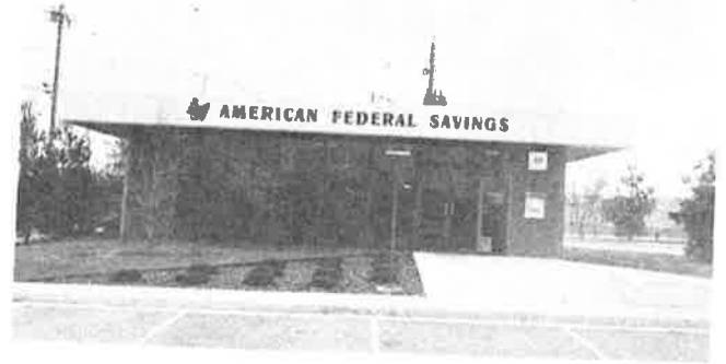
American Federal Savings East First and Trilein Drive
