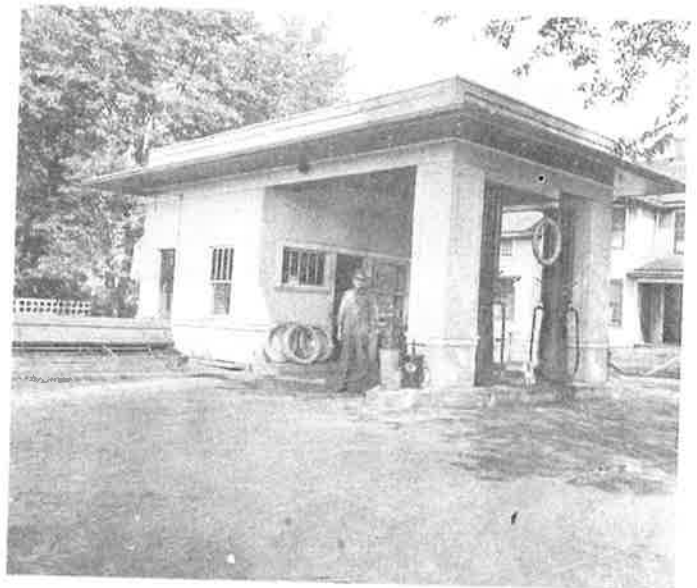
First Filling Station
